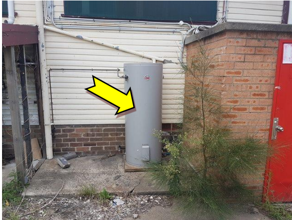
Photo 13. Exterior, north-east elevation, hot water heater – suspected SMF-containing internal insulation.
