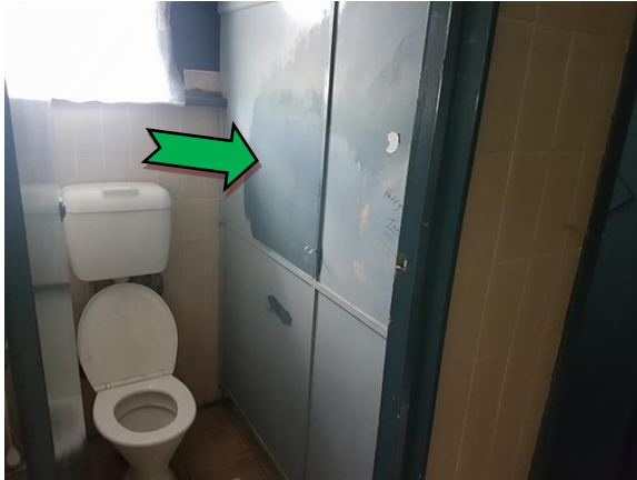
Photo 7. Interior, north-east elevation, toilet, cubicle walls – non asbestos-containing fibre cement sheeting.
