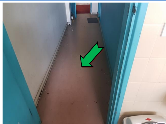
Photo 12. Interior, east elevation, hallway, floor – suspected non asbestos-containing vinyl sheet.
