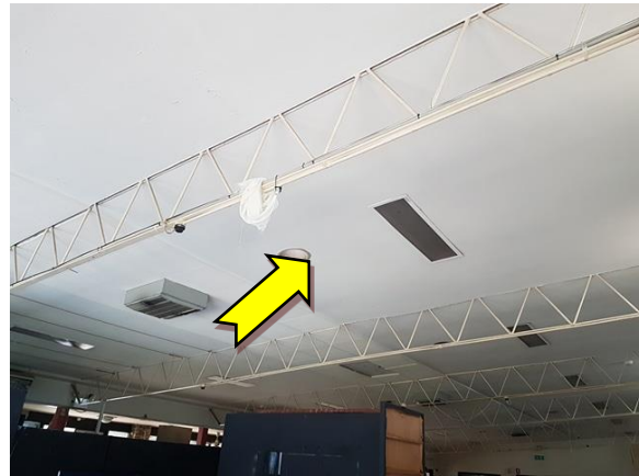
Photo 22. Interior, throughout, ceiling – suspected lead containing white upper coloured paint system.
