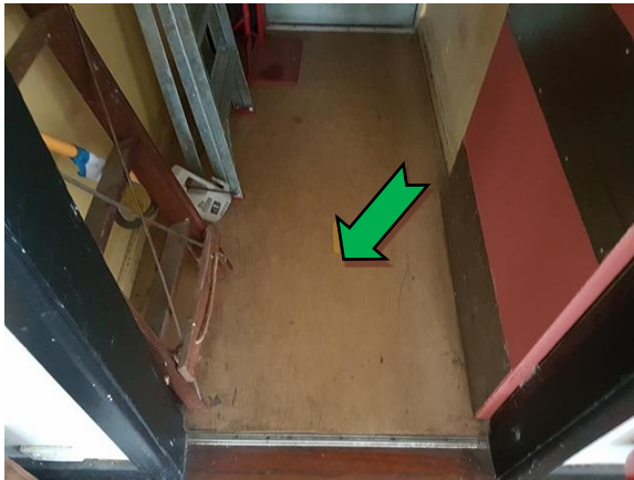
Photo 9. Interior, central east elevation, security room, floor – non asbestos-containing vinyl sheet.
