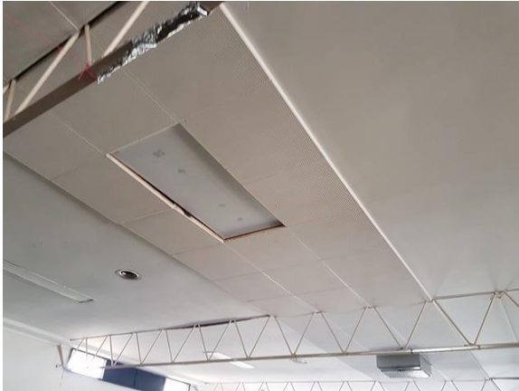
Photo 25. Interior, roof space – no access at time of assessment due to height restrictions.
