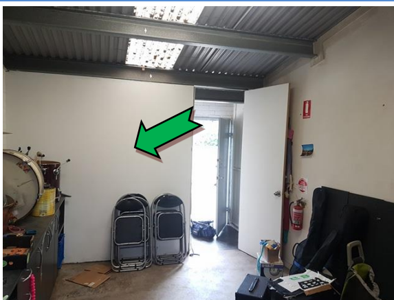
Photo 11. Interior, south-east elevation, garage, wall – non asbestos-containing fibre cement sheeting.
