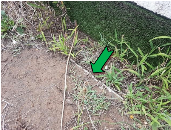
Photo 3. Exterior, bowling green, guttering – non asbestos-containing fibre cement sheeting.
